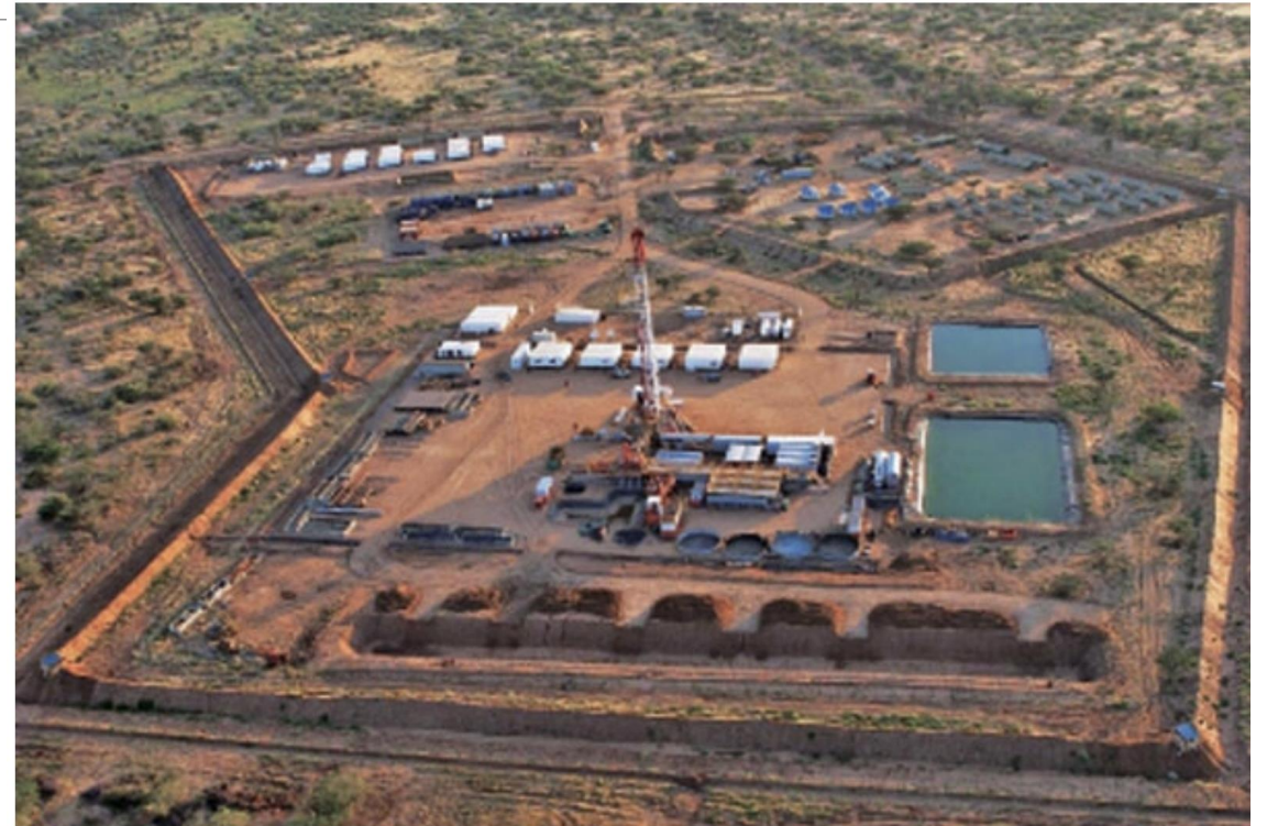
Aerial view of a Tullow oil rig in Turkana County. Turkana Governor Josphat Nanok and Petroleum and Mining Cabinet Secretary John Munyes have asked local residents to allow the Early Oil Pilot Scheme to begin in June as scheduled. PHOTO | FILE NATION MEDIA GROUP
